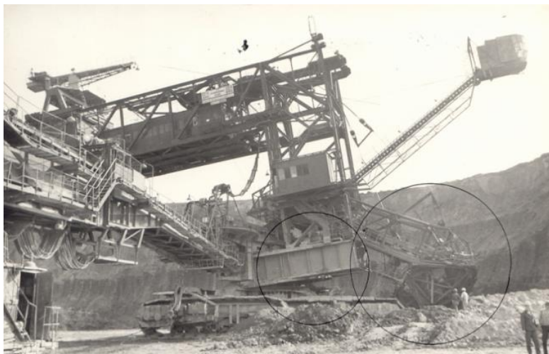
Figure 5. Destruction of SchRs-1200 excavator caused by crack of the wheel boom structure falling-down of wheel excavating boom (drawings before and after catastrophe, picture on-site, dimensions in m) [1]
