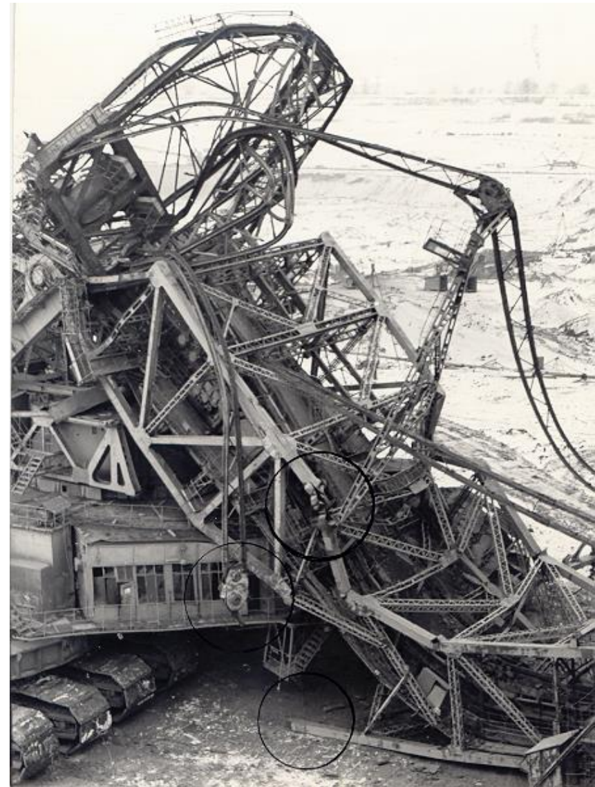
Figure 6. Rapture of one out of two tension members supporting wheel excavating boom of SchRs-1200 [1]
