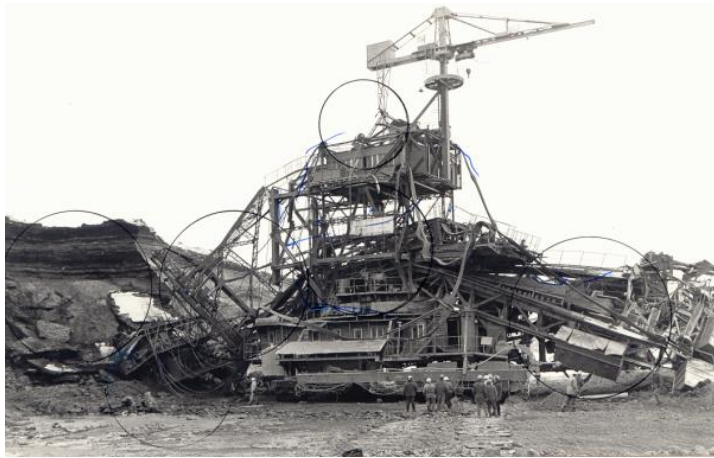
Figure 8. Braking of excavating boom caused by slope creep [1]
