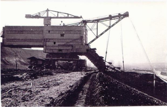
Figure 7. Tilt of chain excavator due to slope sliding [1]
